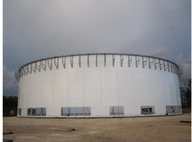
Bolted RTP construction installs in 1/3 the time required for field-weld tank construction.
