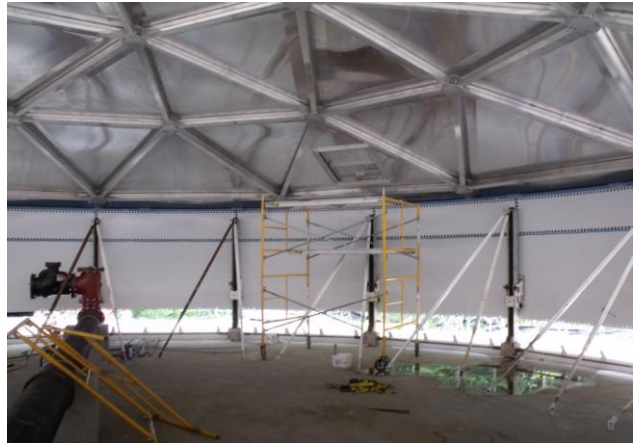
Potable Water with Aluminum Dome
