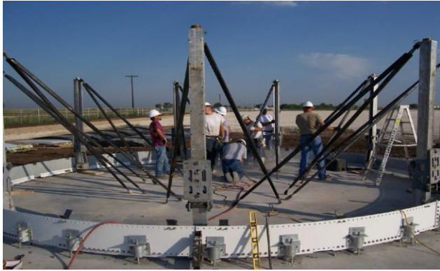
Dry Bulk Tank – Base Anchor Ring
