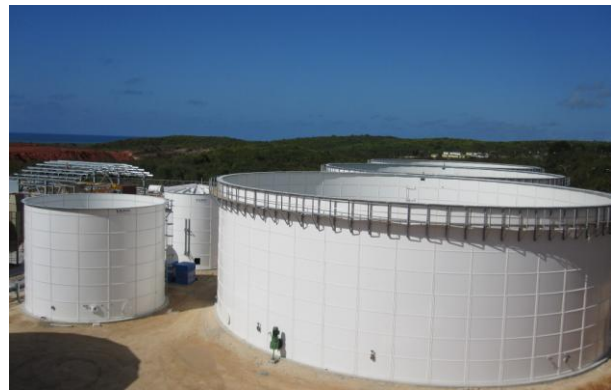
Anaerobic Digester Tanks
