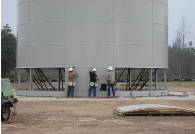
Dry Bulk Hopper Tank
