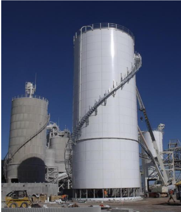
Bolted RTP construction installs in 1/3 the time required for field-weld tank construction.
