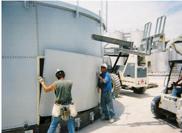
Dry Bulk Panel Installation
