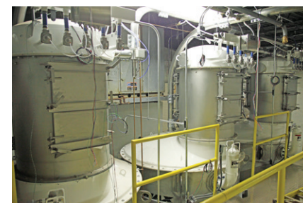
Vac-U-Max pulse dome filter covers above vacuum receivers equipped with side access doors
