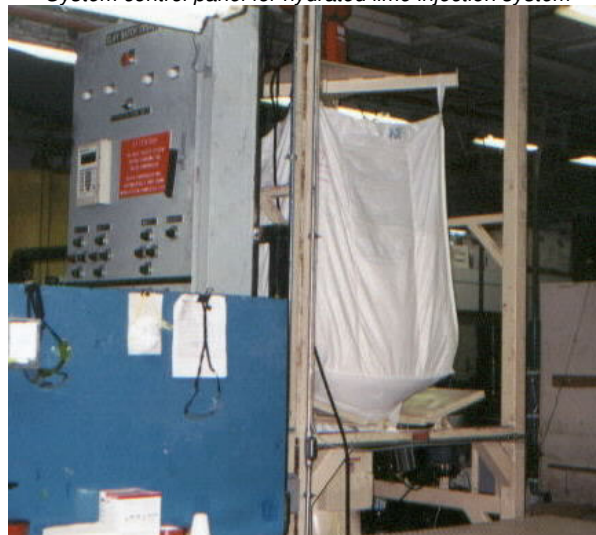
Bulk bag unloader and system controls for kaolin clay feed system
