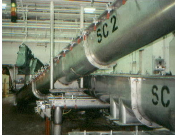
Soft Sugar distribution system conveyors
