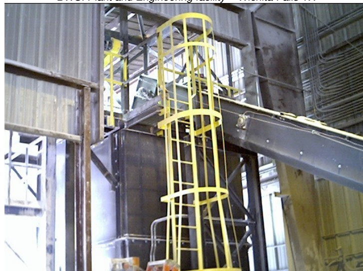
Waste gypsum handling system with drag conveyor, bucket elevator, and hopper
