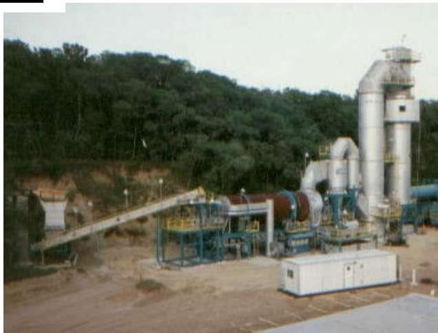
Hazardous soil remediation system for kiln feed and ash discharge
