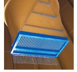
A lined, steep slope chisel bottom hopper promotes coal flow and reduced the tank height requirements. Come to Tank Connection for recommendations, innovations and custom designs.
