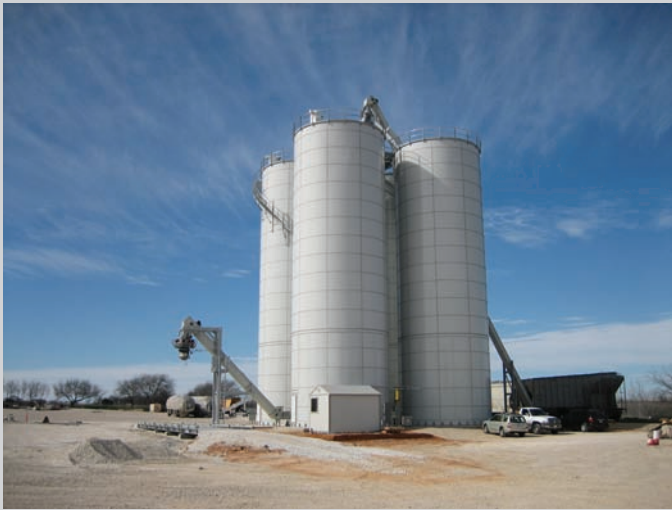
RTP (rolled, tapered panel) bolted design
