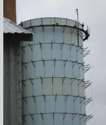
API 12B flanged panel tank - scaffold built
