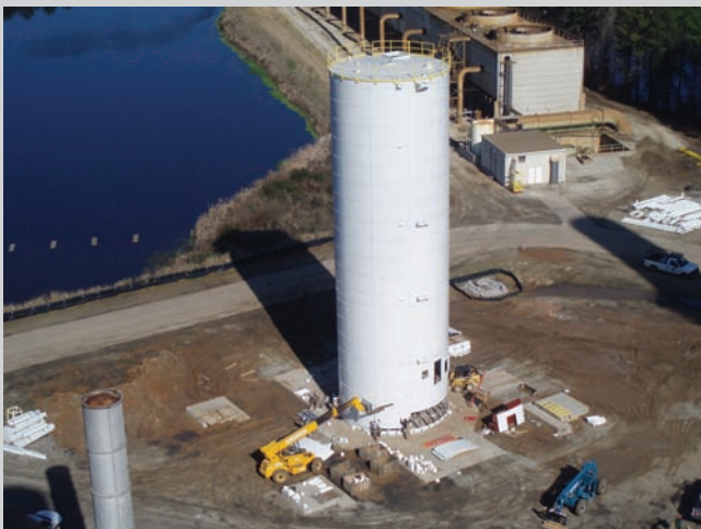
RTP dry bulk silo under construction
