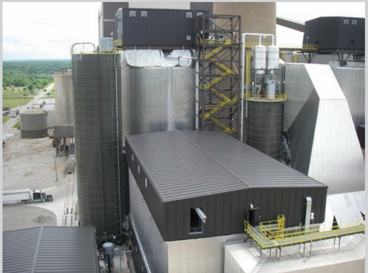
Power Utility - Lime & Ash Storage
