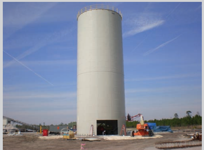
Field installation at grade level utilizing synchronized jacks
