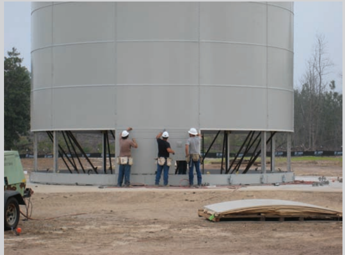
RTP Tank under construction
